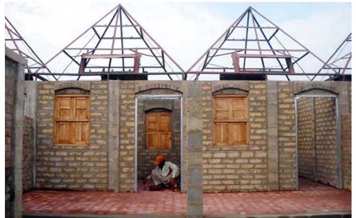
Energy efficient, environmentally sustainable houses being constructed in Pakistan. Photo: Masood Lohar
