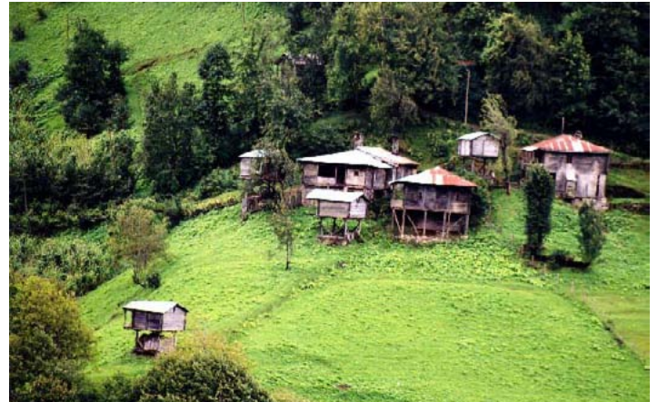
Insulated wooden houses, Turkey. Photo: SGP Turkey
