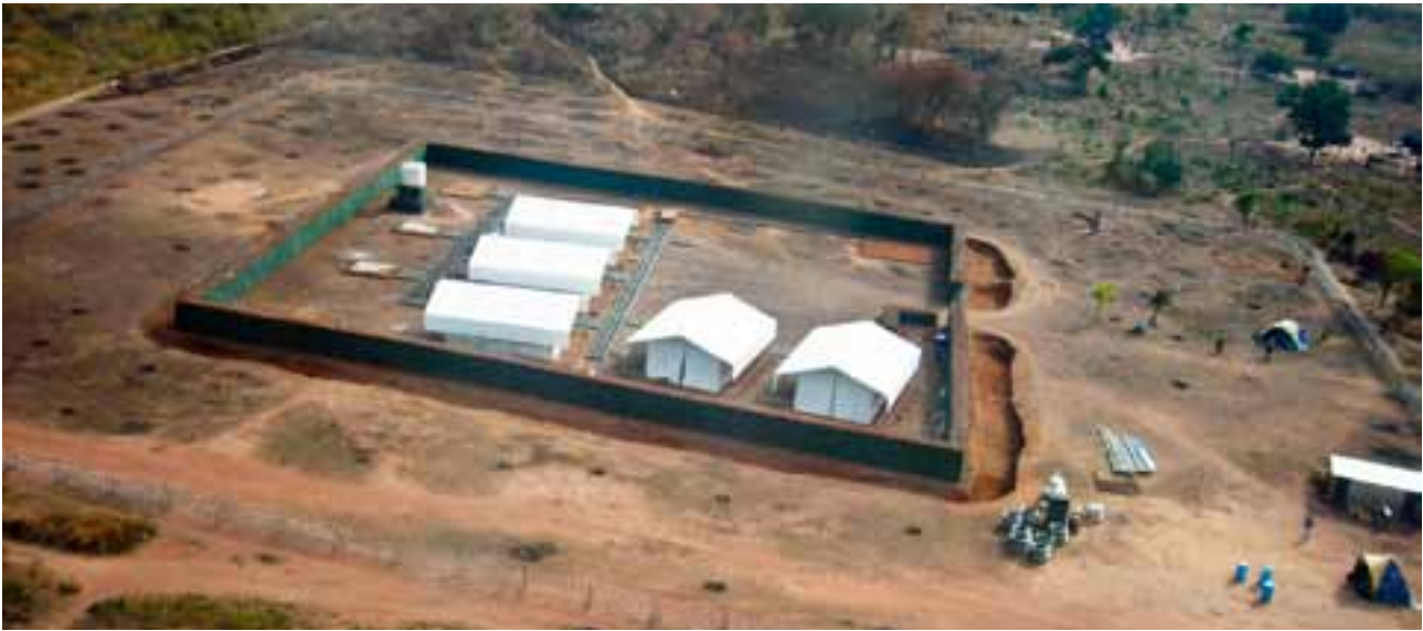
A referendum support base constructed by UNOPS on behalf of the United Nations Mission in Sudan as part of preparations for the January 2011 referendum in Sudan. Photo: UNOPS
