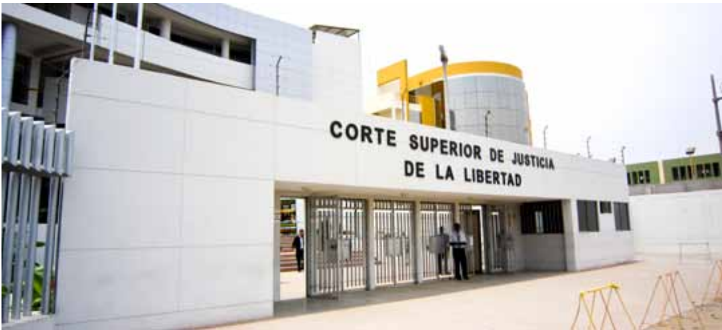
The High Court of the Peruvian district of La Libertad, part of an infrastructure project implemented by UNOPS on behalf of the Peruvian Judiciary and UNDP. Photo: UNOPS/Aida Arifo-Fernández
