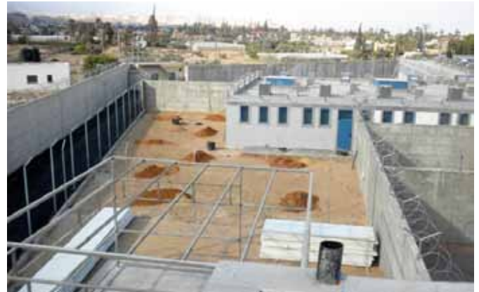
Construction of the Jericho prison underway
