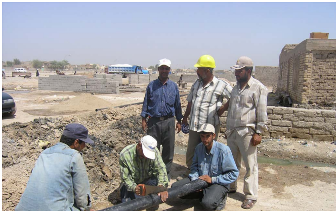
New water piping as part of the Six Water Networks Iraq
