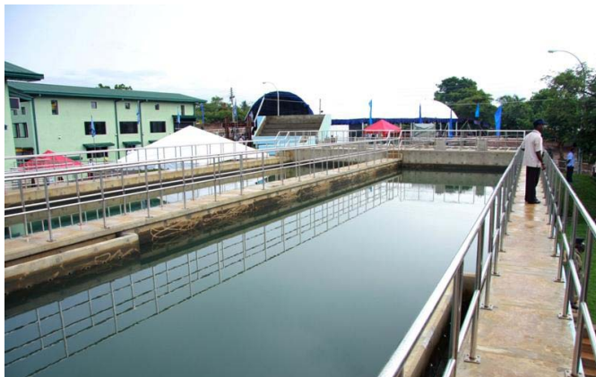
Sedimentation tank in Tangalle, Sri Lanka
