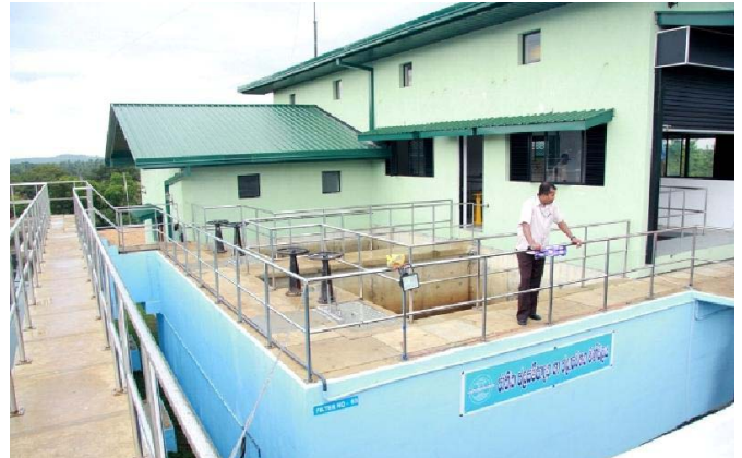
Treatment plant for the Tangalle supply scheme, Sri Lanka
