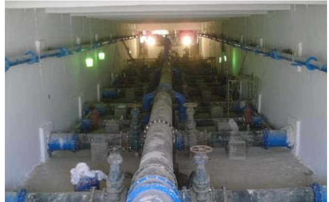
Rehabilitated piping system in Kerbala, Iraq
