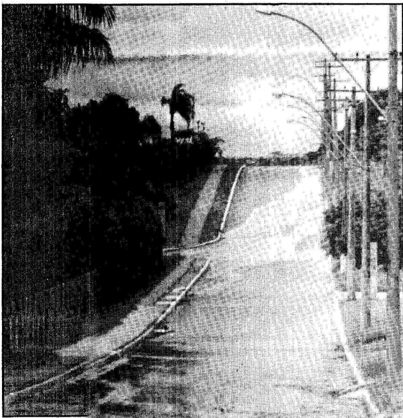
Com as chuvas, as fossas transbordam e o esgoto corre pelas ruas
