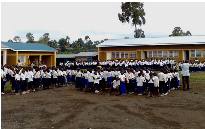
New buildings at Biayi Public School, DR Congo, constructed by UNOPS as part of a World Bank rehabilitation project.
