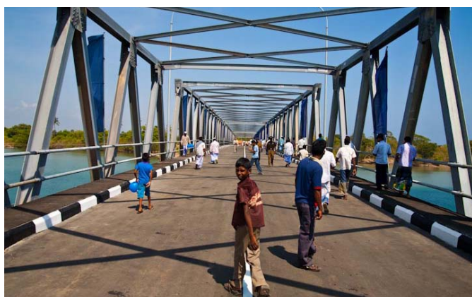
Irrakandi bridge, Sri Lanka, restored with Government of Spain tsunami funding with UNOPS as implementing agency.
