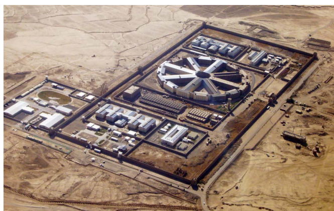
Finished prison at Pol-e-Charkri, Afghanistan, funded by Government of Italy and partly rehabilitated by UNOPS.
